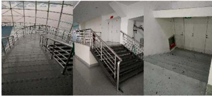
Fig. 5. Schematic diagram for design defects of exit of stand d, e and f
